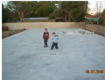
The freshly laid slab on which Stepping Stones will stand
